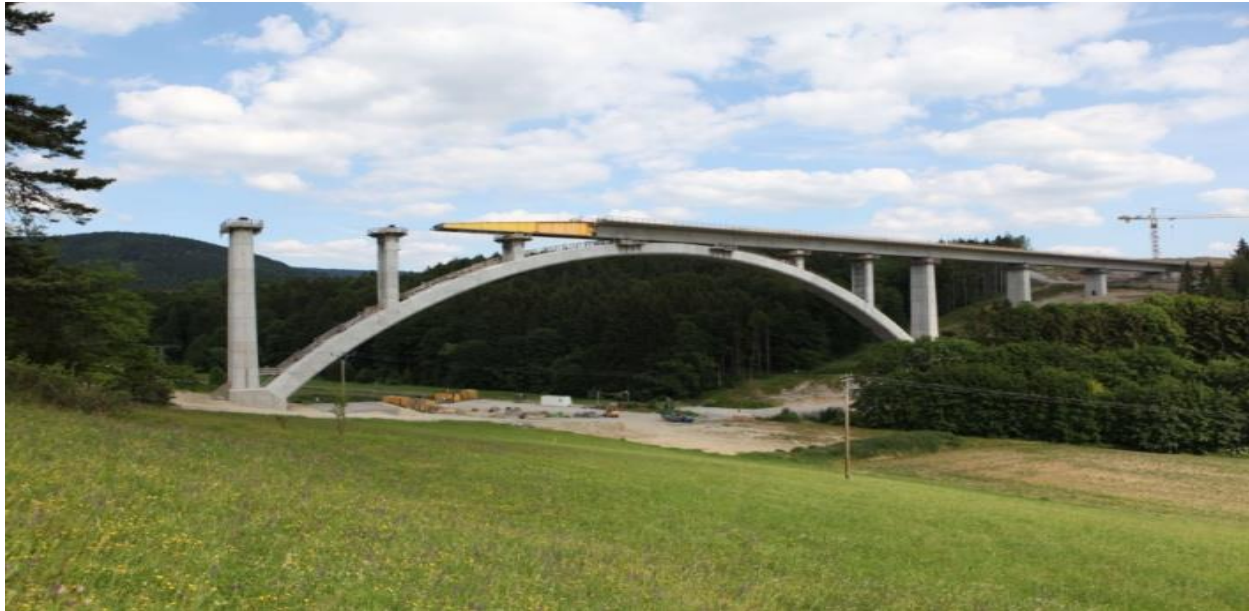
Fig. 1 Incremental bridge launching [1]
