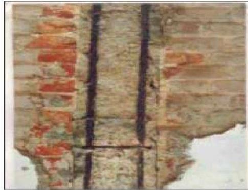
Fig No. 4.4 (a) Corrosion of Reinforcement
